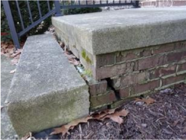
Step on front stoop separated
